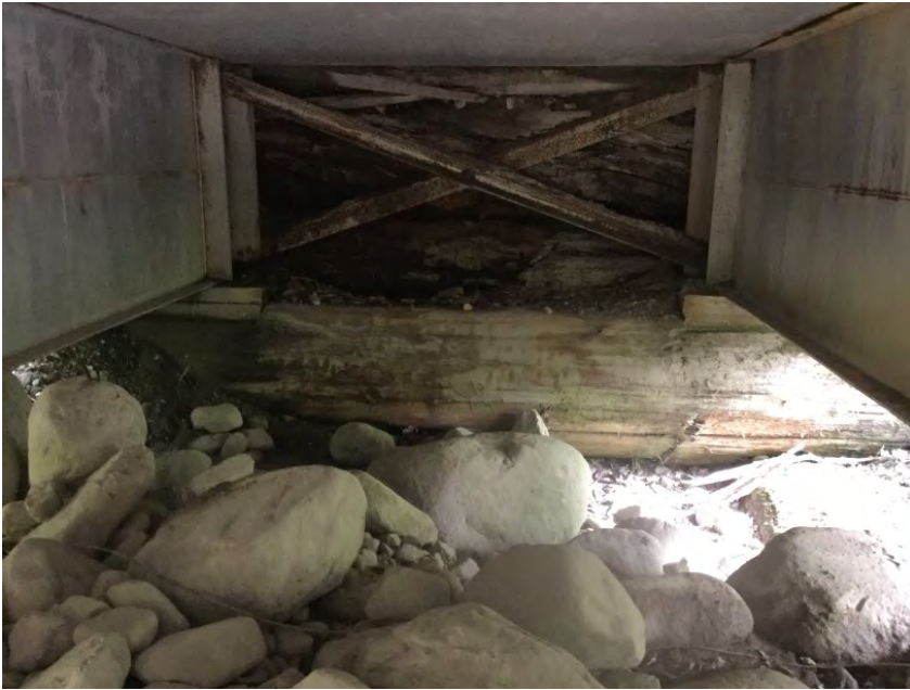
Left Bank Abutment when facing downstream
