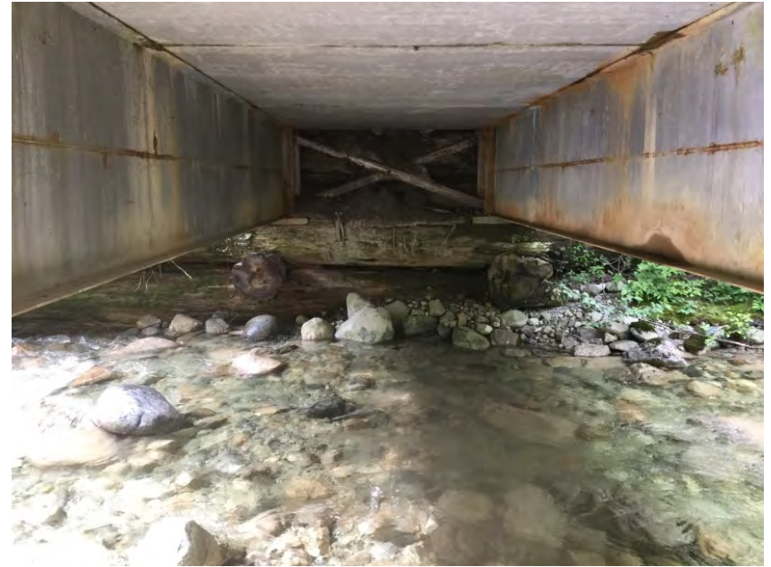
Right Bank Abutment when facing downstream
