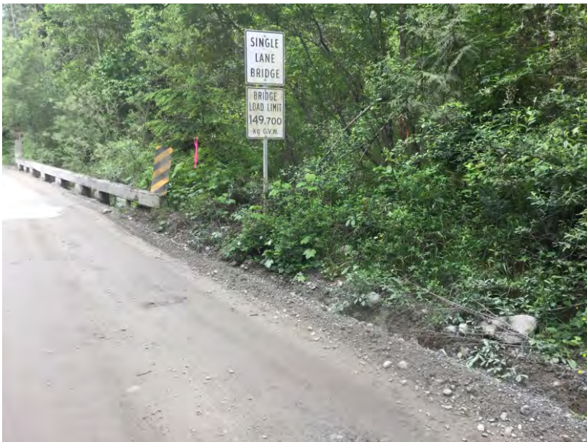
Missing left upstream fender
